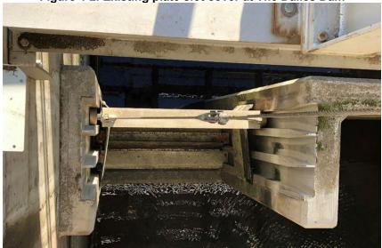
Figure 4-2. Existing plate slot cover at The Dalles Dam
